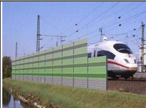
Full-height noise barriers are defined in this factsheet as being barriers greater than 1.0m in height. When used on railways, these barriers are installed at the trackside, generally no closer to the track than the signal posts, electrification masts, etc. and are one of the most common forms of noise mitigation used on railways.
