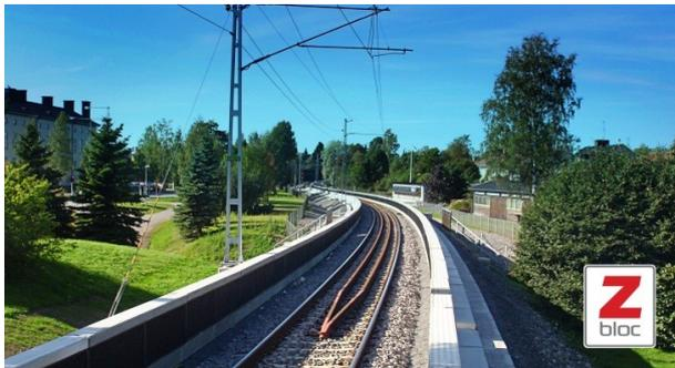
Low-height noise barriers are defined in this factsheet as being less than 1.0m high). When used on railways, these barriers are located at or in very close proximity to the ends of the sleepers (typically ~1.7m from the centreline of the track) and provide an alternative to conventional full-height barriers at the trackside, screening noise in close proximity to the source.
