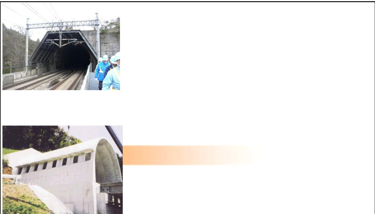
The most common materials used for tunnel hoods are concrete and steel (Saeki and Watanabe, 2008), see for example Figure 4, with concrete structures generally used on
