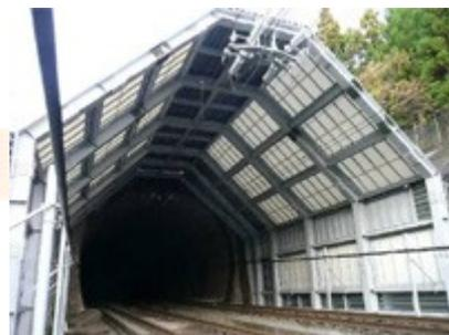
(b) Tunnel hoods made with lightweight membrane panels (Photo: East Japan Railway Company)
